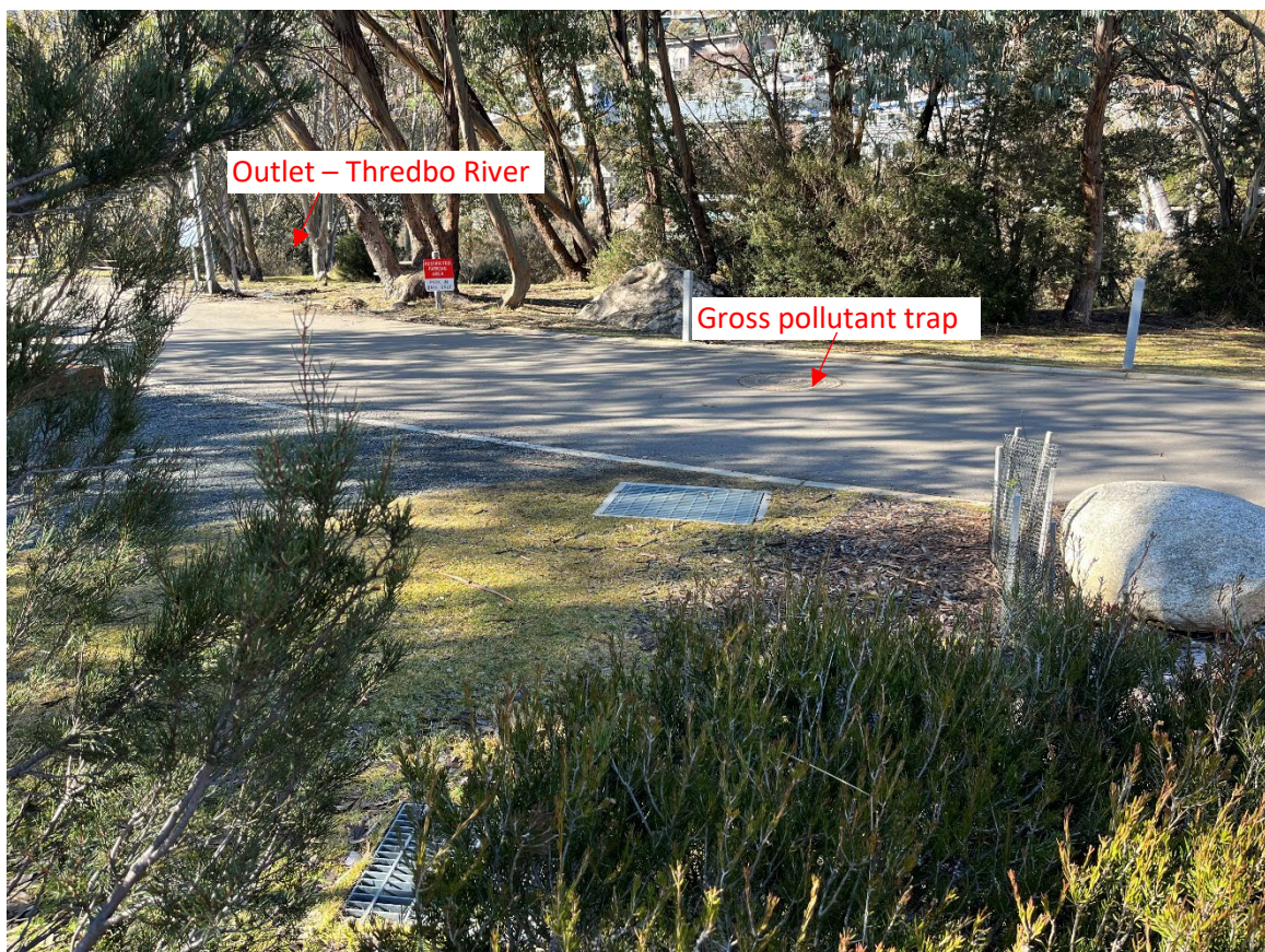
Photo 5: existing drains between Gondola and road - feed into GPT
