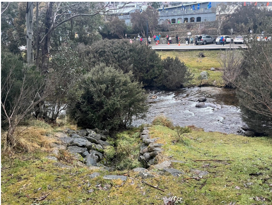
Photo 3: Outlet into thredbo River (existing rock headwall)
