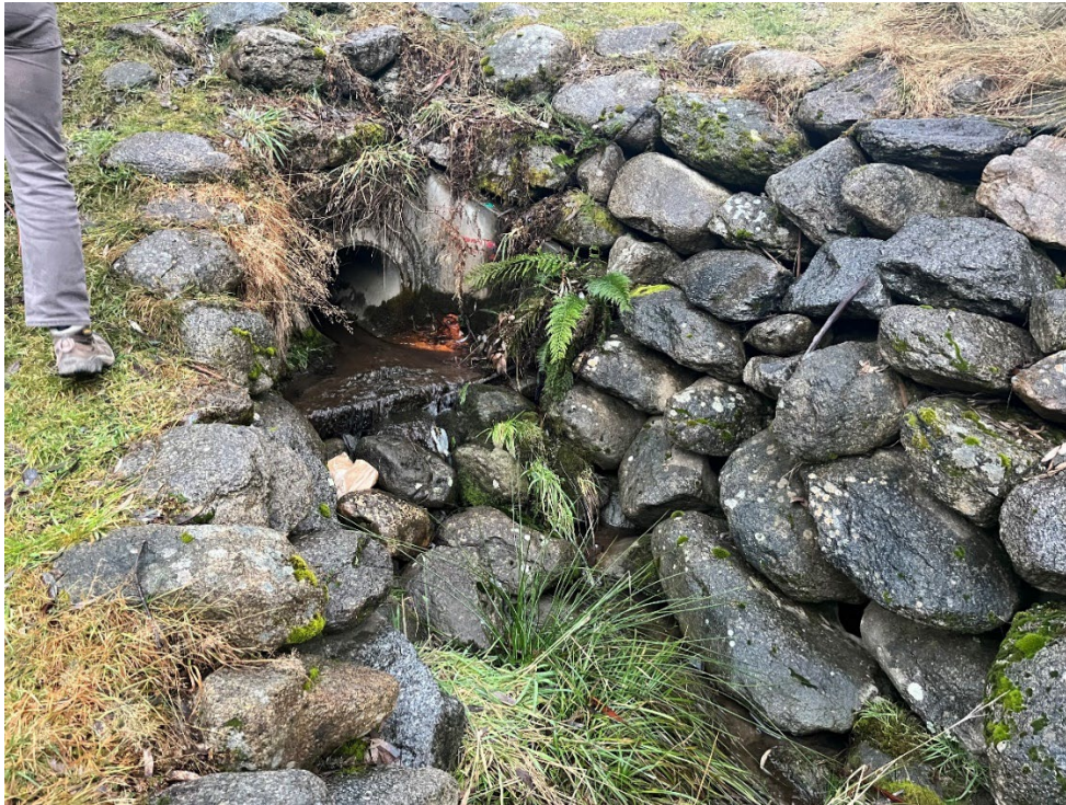
Photo 2: Existing rock headwall, outlet to Thredbo River (GPT piped to outlet)
